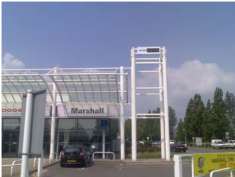
Left and above: 300mm character height yellow LED outdoor clock one of a pair using master controller. Mounted on steel tower
